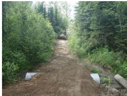
Culvert being installed
