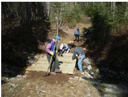
Installation of a bridge
