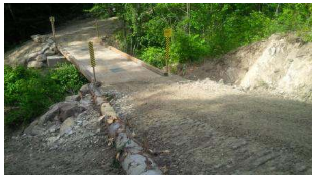
New Bridge on Burgess Trail
