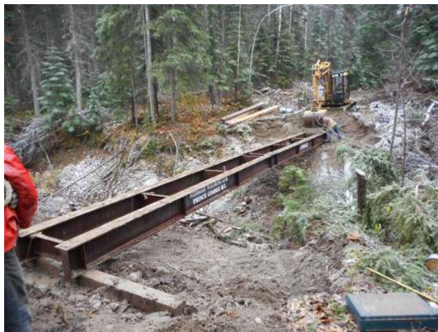
Bridge girders being installed
