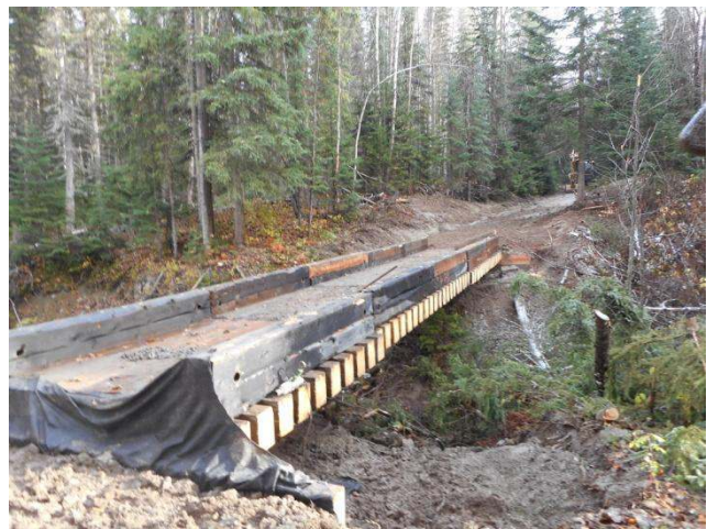
Decking installed on the girders
