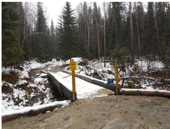
Bridge installed, minor work on approaches needed
