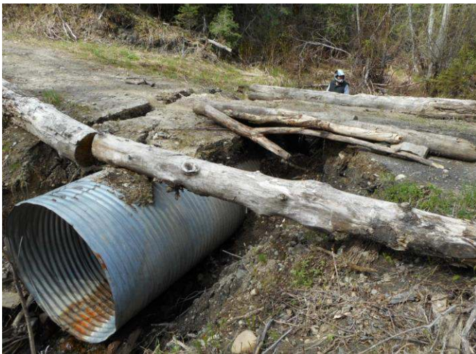
George's Dip culvert washout
